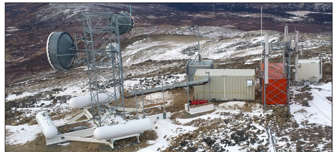
A new communication site is completed on Bald Mountain in 2016.
